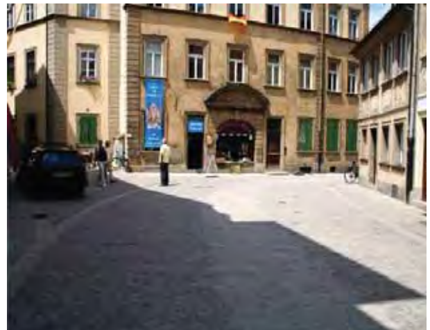
The Sandstrasse, where smooth setts are used in the centre of the street with rough tumbled setts either side
