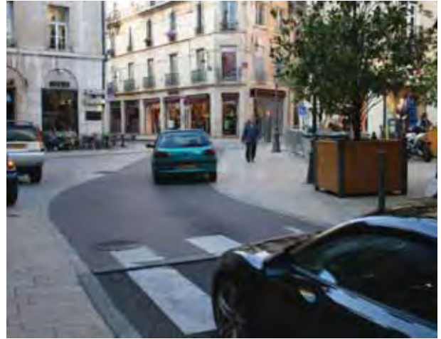
Bringing the road up to the pavement level with a bump!
