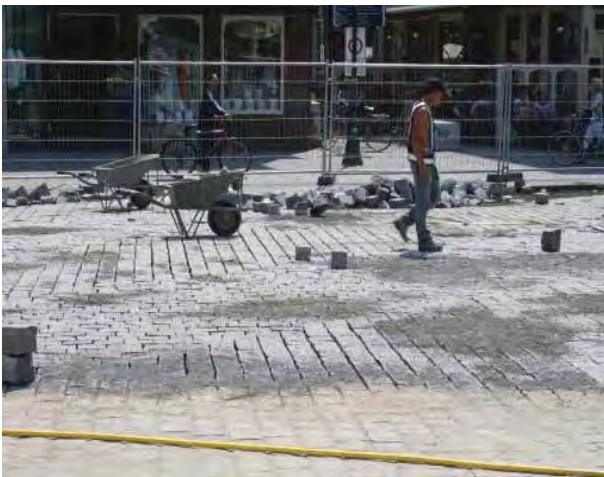
Laying granite setts in the Market Place
