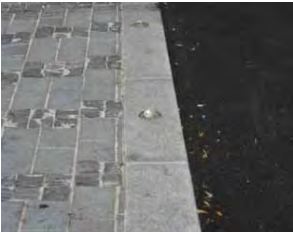
In this part of the city, lights are used to define the kerb line
