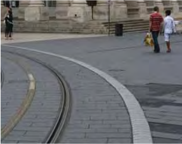
Note the raised metal divider between the tram line and pedestrian area
