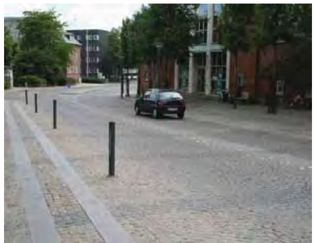
Centre of the carriageway defined by studs and smooth slabs used to assist in pushing buggies and for cyclists
