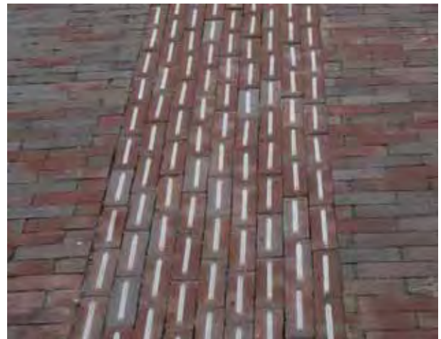
Defining the join between cycleway and footpath
