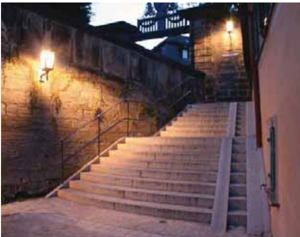
Lighting plays an important role. Note the ramp to help cycles to be pushed up and down the steps
