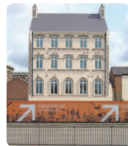
St Burnett House, Hull: before & after phase I of work. Phase II is scheduled for 2007
