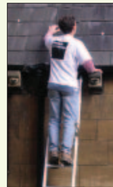
Regular inspection is the key to systematic maintenance.
