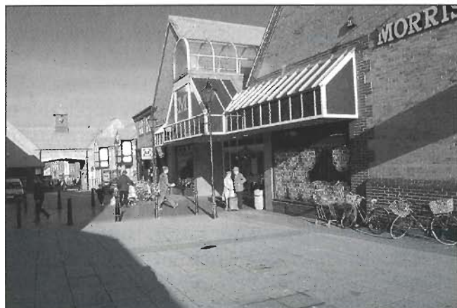
Town centre foodstore, Newark
