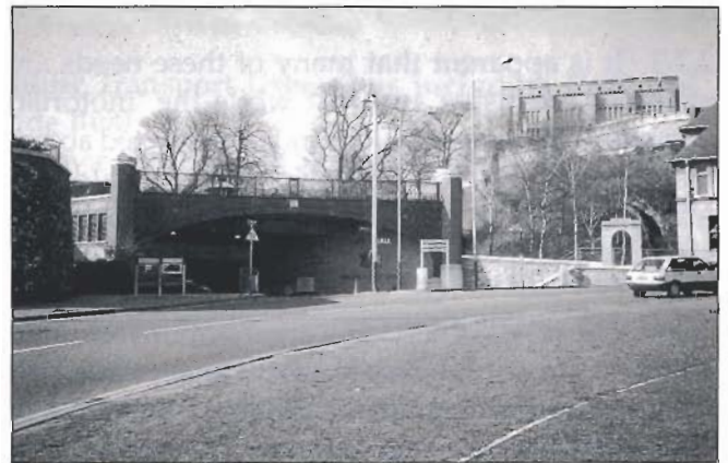
Entrance to underground servicing and car parking at Castle Mall in Norwich
